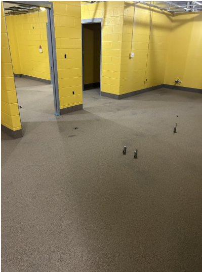
Installing resinous flooring on level 2.
